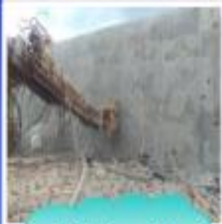
Soil Nailing Work
