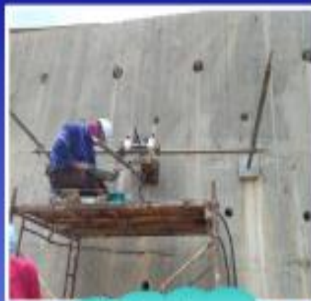
Pull Out Test for Soil Nail
